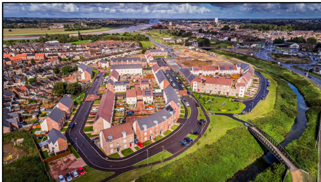
Aerial view of Nar Valley Park
