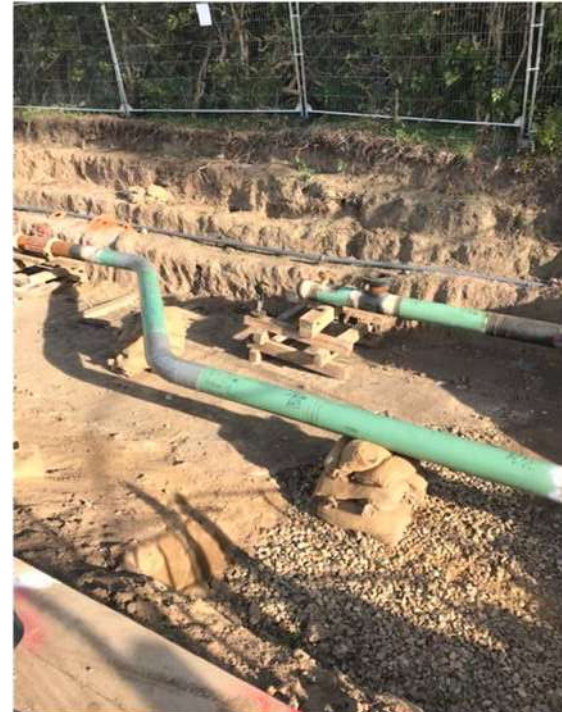
Relocation of gas main
