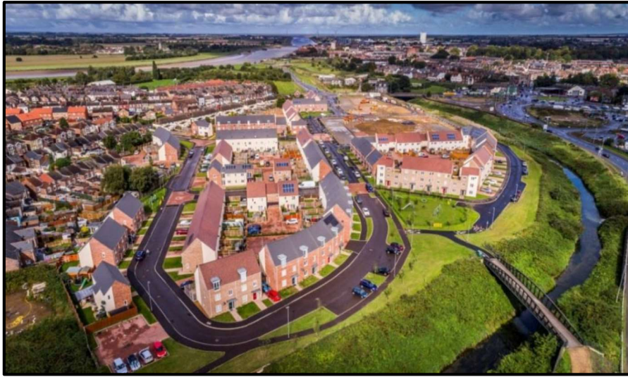
Aerial view of Nar Valley Park
