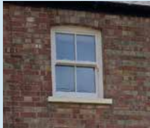
Sash window and details
