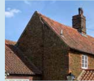
Gabled roof and red pantiles
