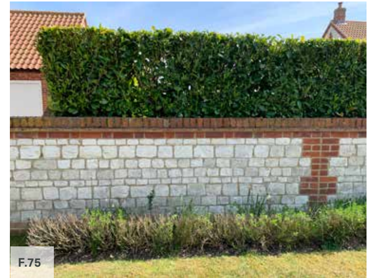
Figure 73: Low wall built with red brick and clunch on Docking Road
