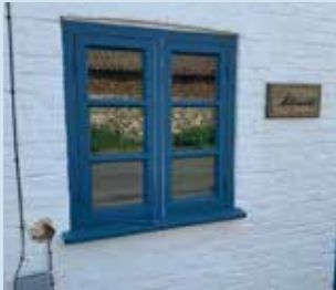
Casement window with painted timber
