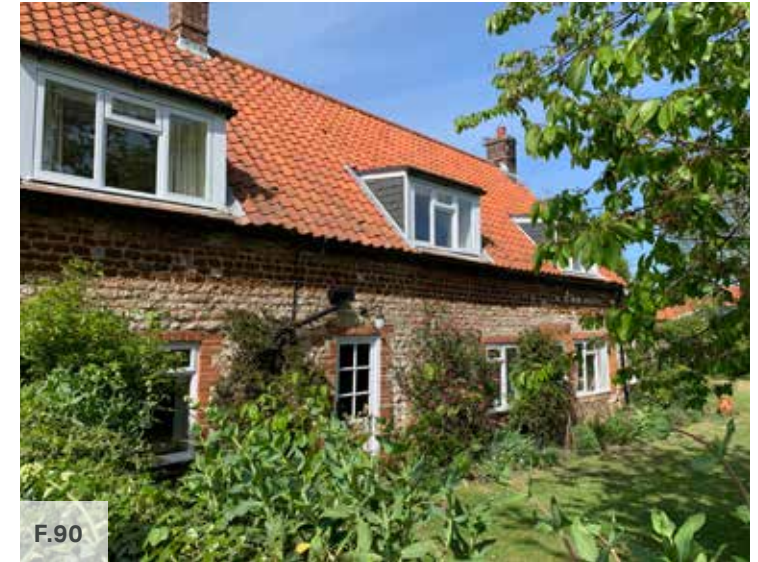
Figure 88: Mix of carrstone and red brick on wall and use of red brick as decoration around casement windows
