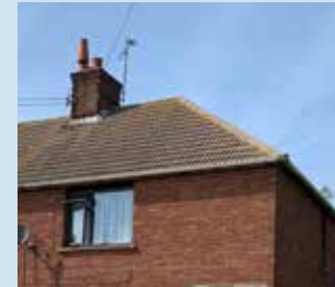
Hipped roof with concrete tiles
