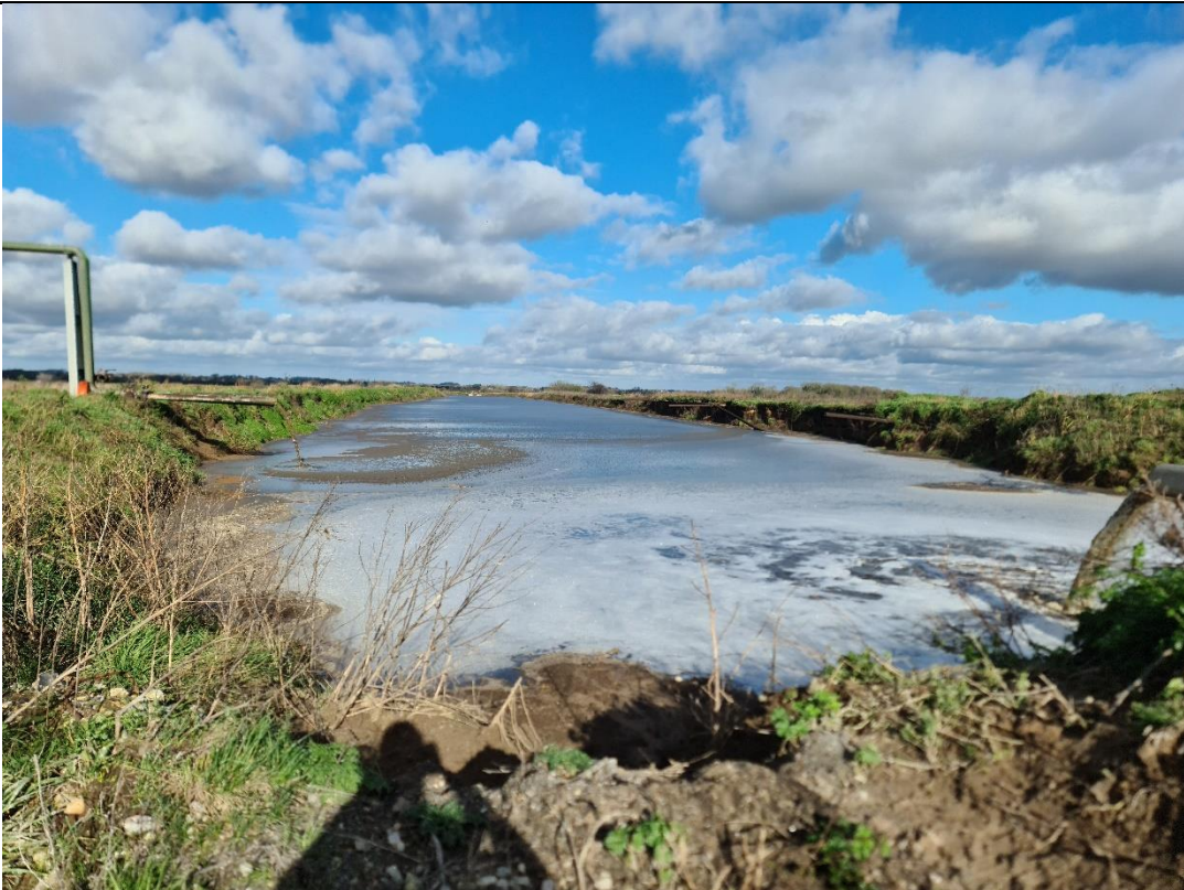
Photograph 6: Secondary initial settlement bed with material flowing in.
