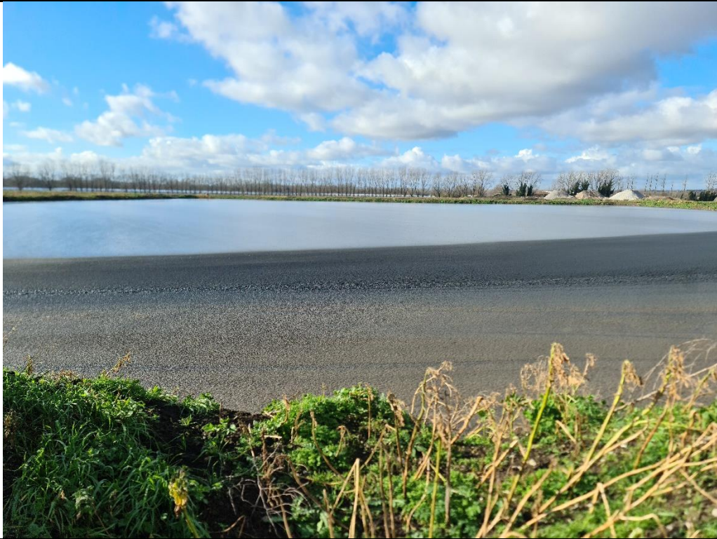
Photograph 3. Finer material in a adjoining settlement tank.
