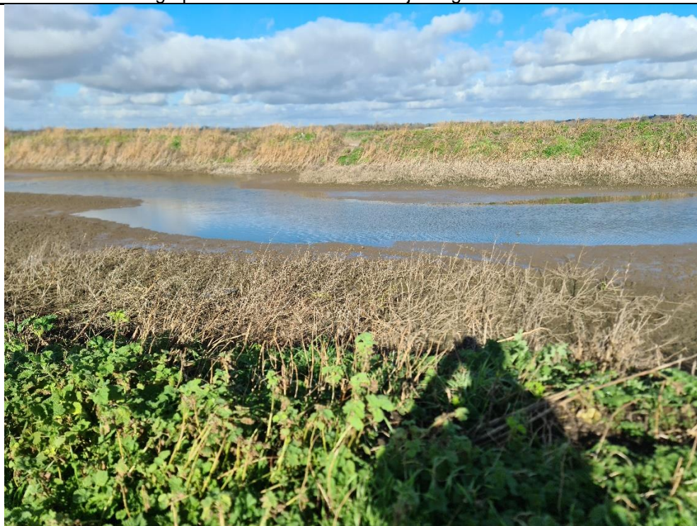
Photograph 4. Heavy deposition in a settlement bed on the north of site.
