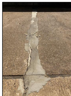
Concrete repair to promenade
