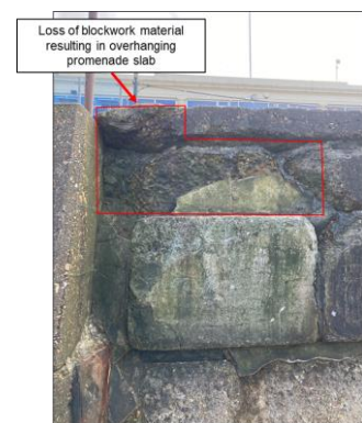
Concrete repair to seawall
