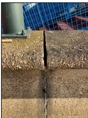
Sealant replacement to wave-return wall
