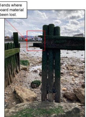
H&S cutting pointed edges of timber groyne element flat.
