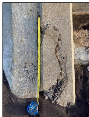
Concrete repair to seawall
