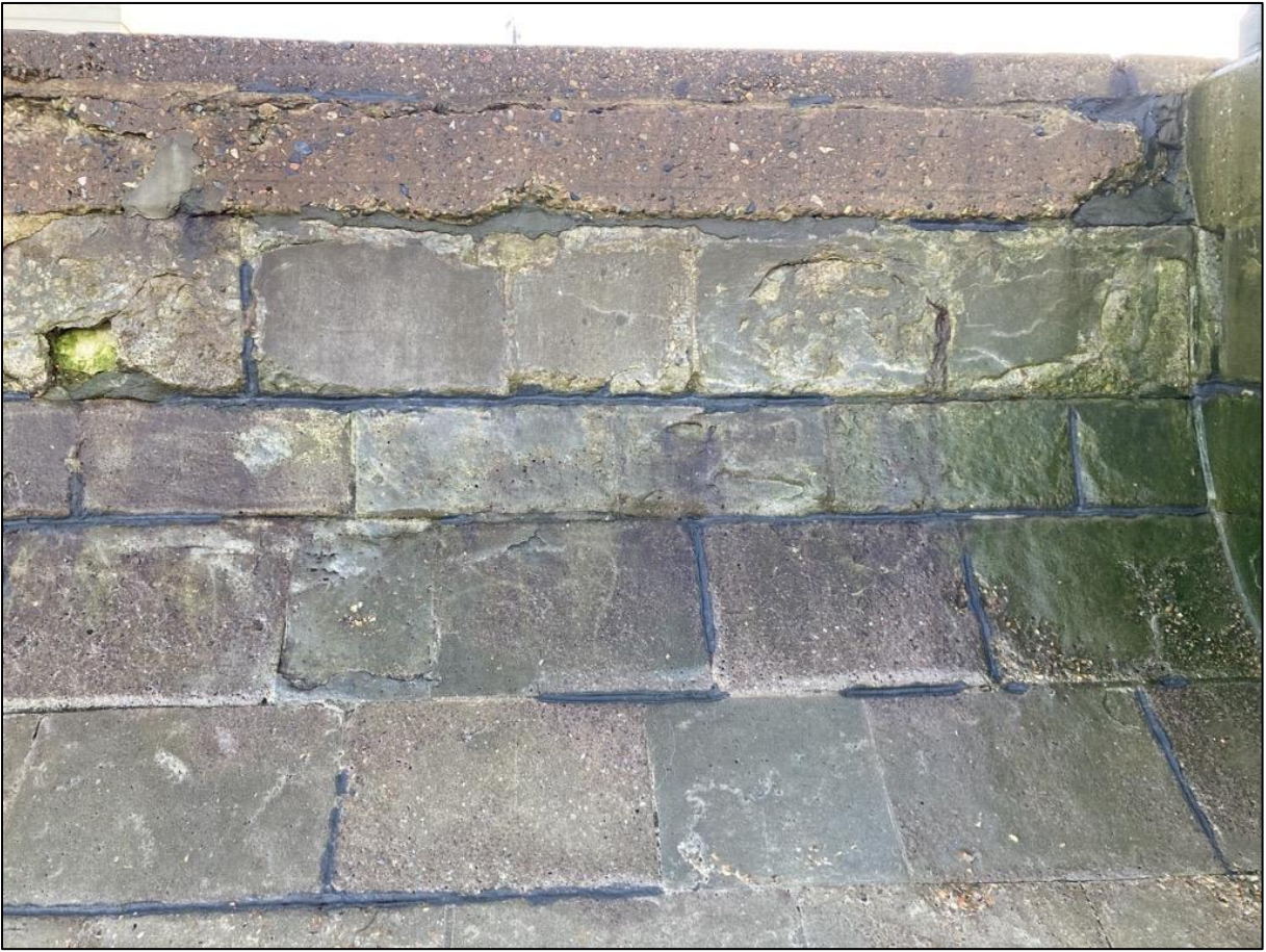
Blockwork seawall after repair mortar joint replacements
