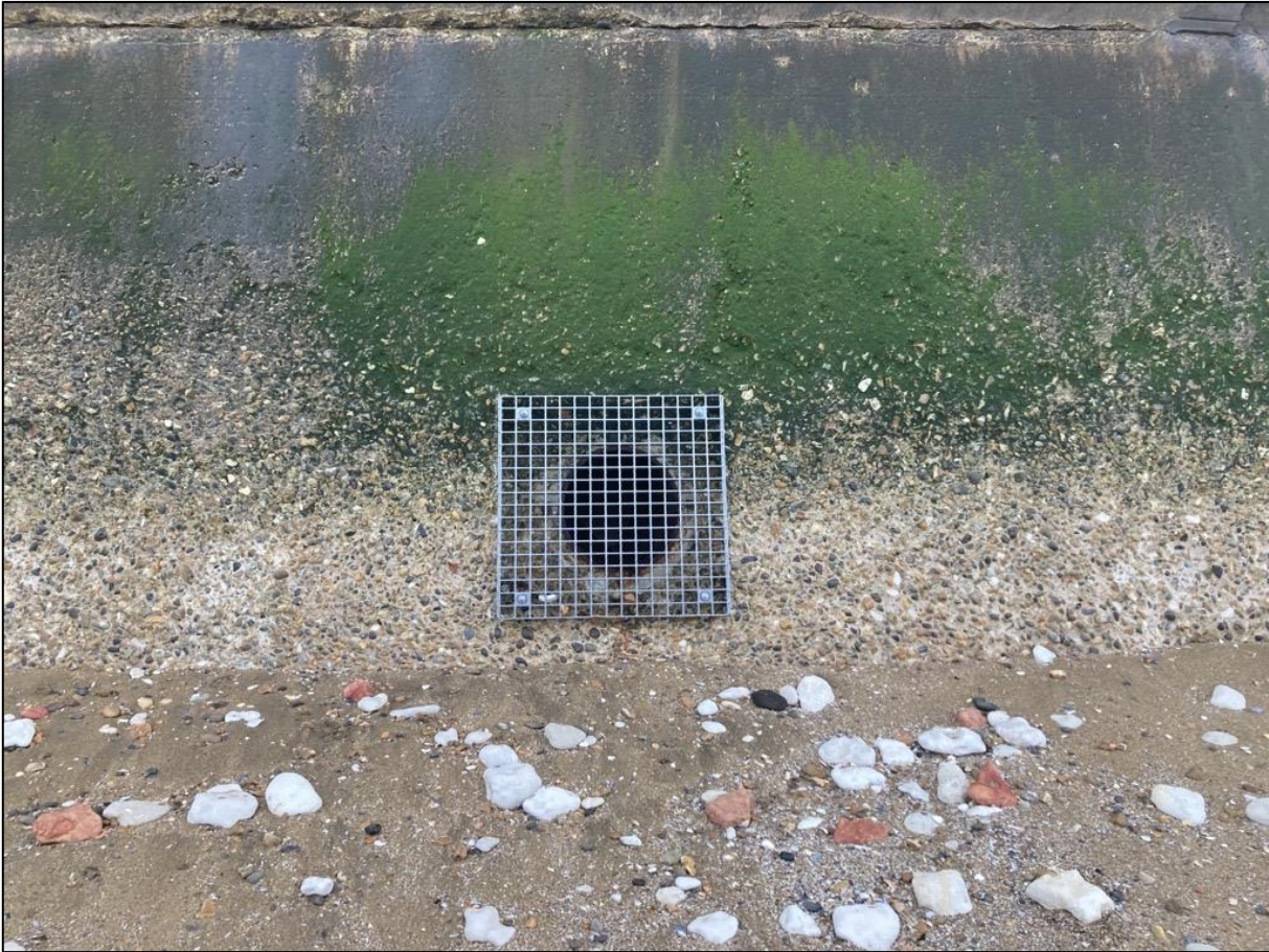
Replaced outfall cover
