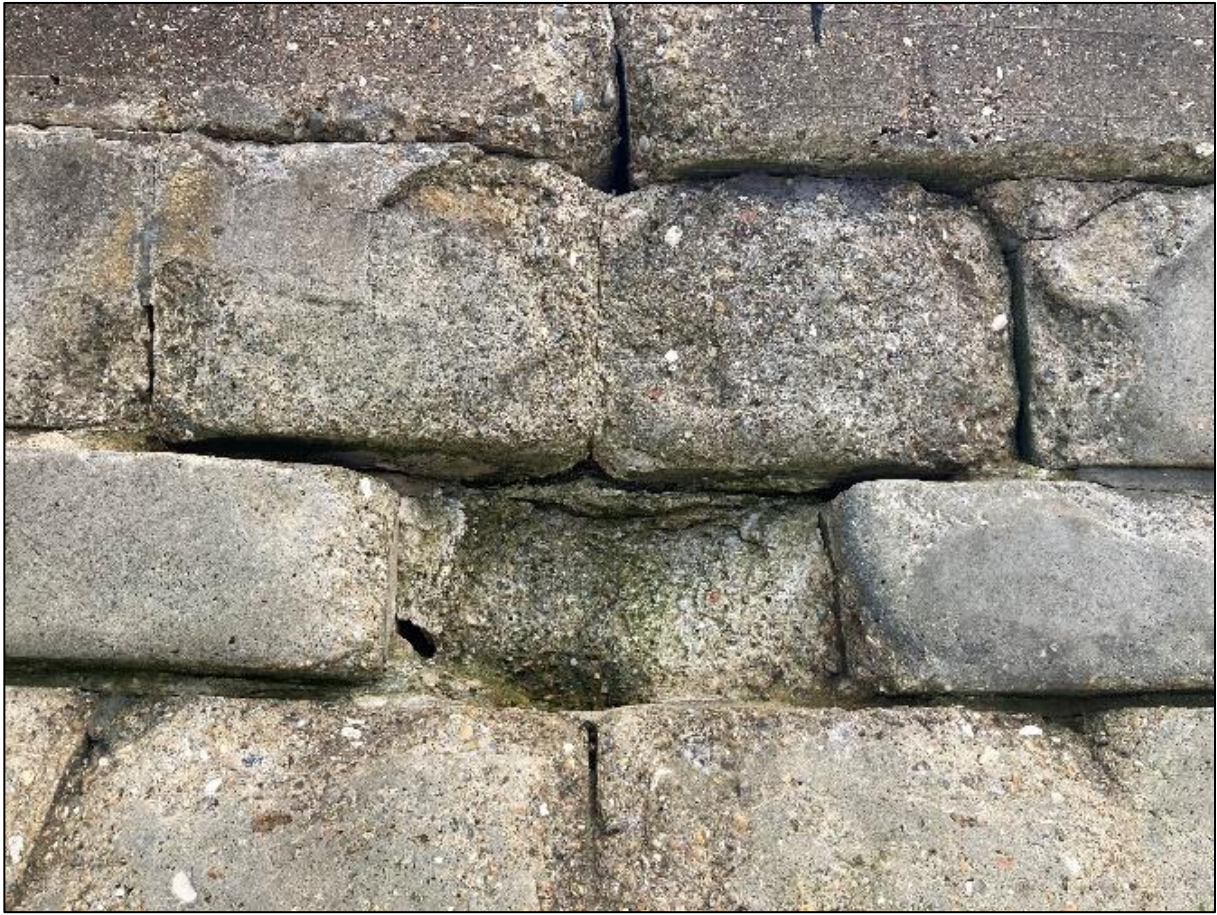
Blockwork seawall before mortar joint replacements
