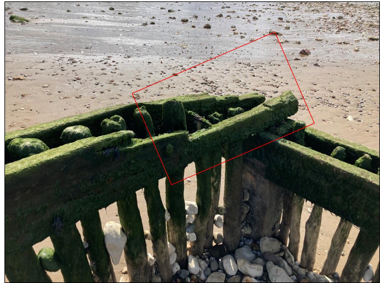
Additional fixings required to secure timber groyne element
