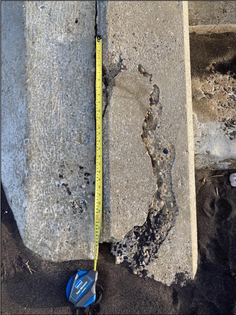
Concrete patch repair required to seawall
