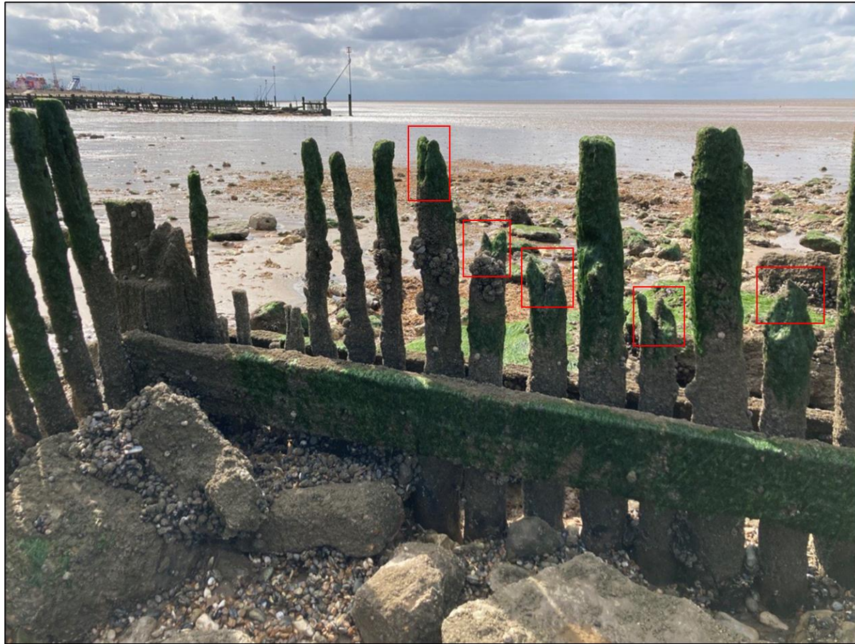
Cutting flat of pointed timber groyne element required
