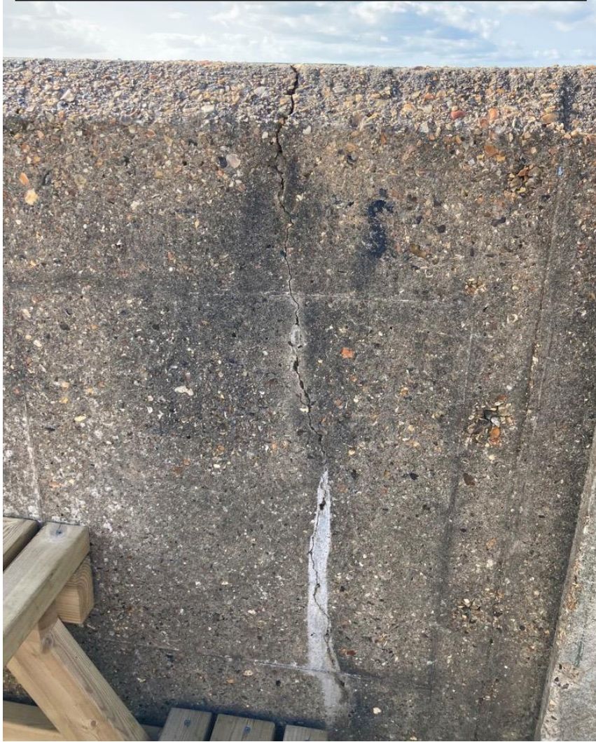
Wave-return wall before concrete patch repair
