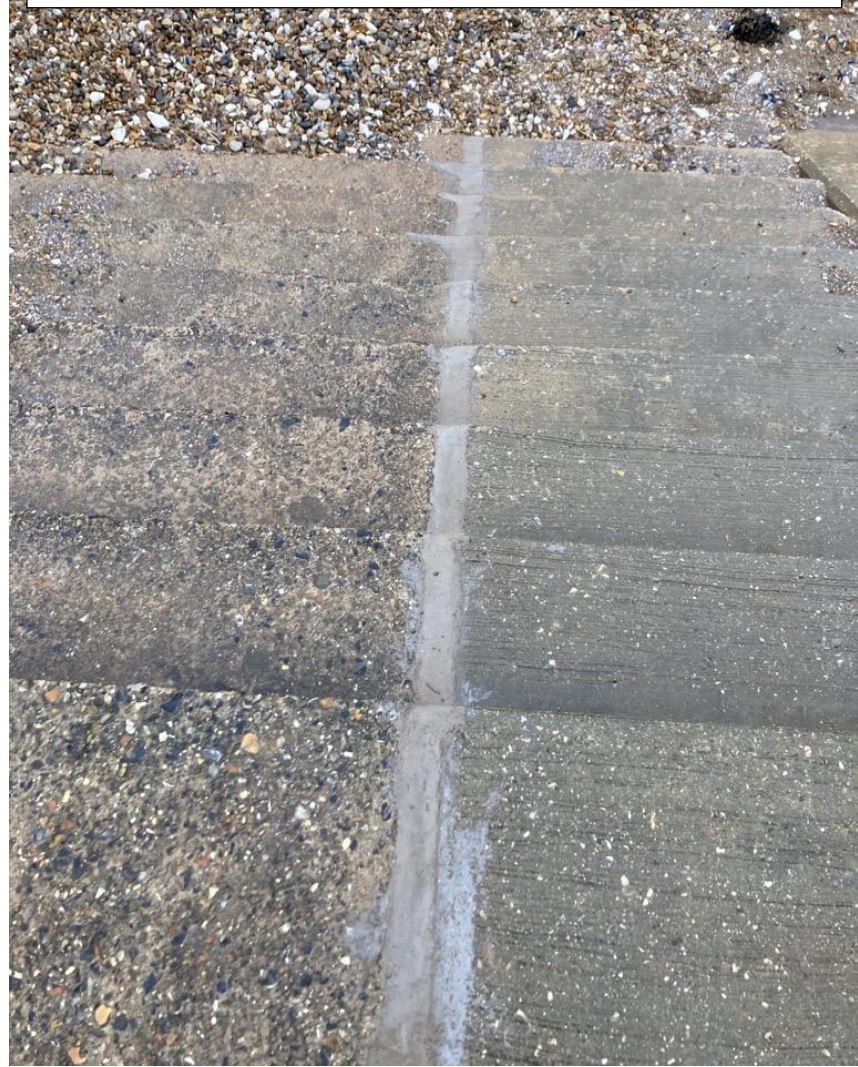
Wave-return wall after mortar joint replacement
