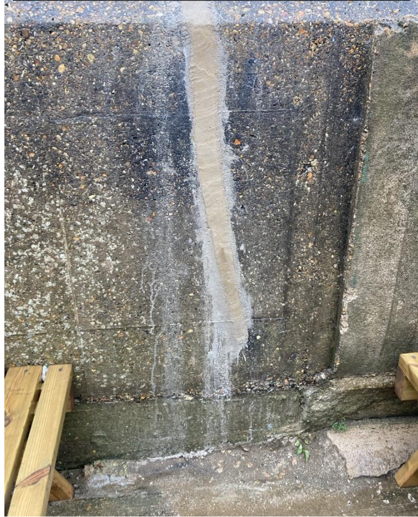
Wave-return wall after concrete patch repair
