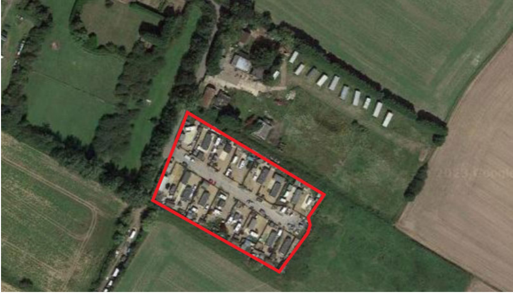
Fig. E - Location of West Walton Court, Blunts Drove (Public Gypsy Traveller Site)
