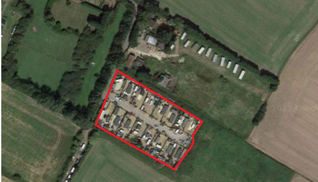
Fig. E - Location of West Walton Court, Blunts Drove (Public Gypsy Traveller Site)
