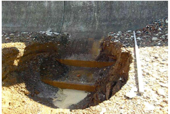
Trial pit undertaken at base of Hunstanton seawall in 2012.
