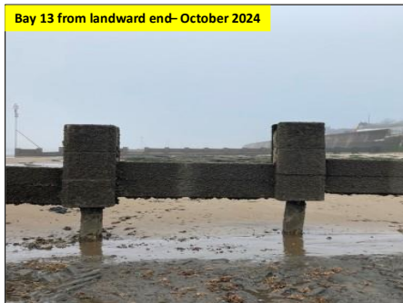
Top two horizontal concrete planks removed
