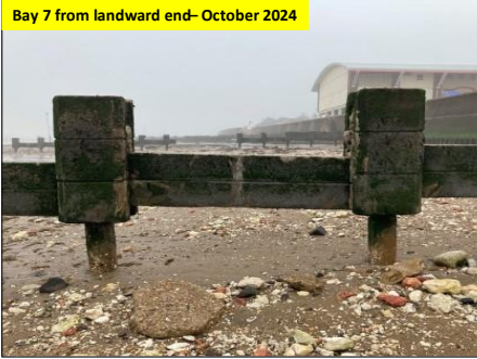
Top two horizontal concrete planks removed
