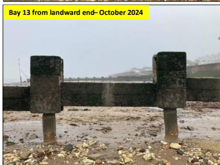
Top two horizontal concrete planks removed
