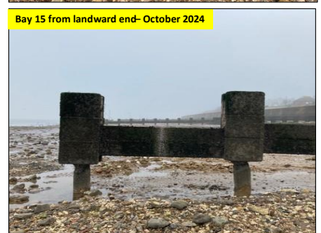
Top two horizontal concrete planks removed
