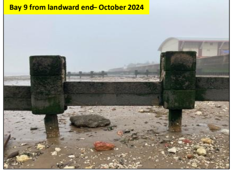
Top two horizontal concrete planks removed
