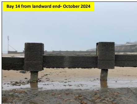
Top two horizontal concrete planks removed
