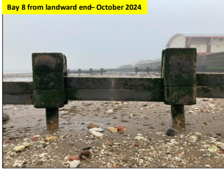
Top two horizontal concrete planks removed
