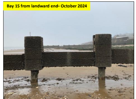
Top two horizontal concrete planks removed
