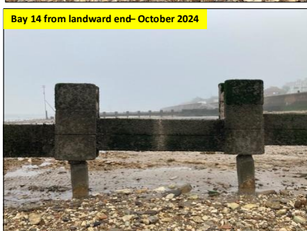
Top two horizontal concrete planks removed
