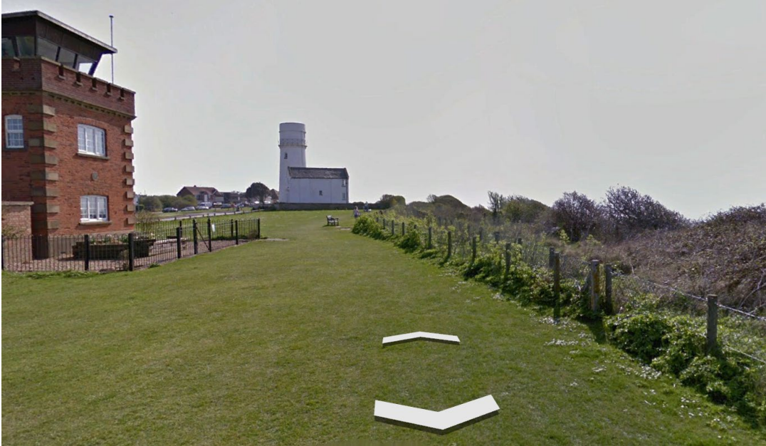
Figure 51 = View of fence line from Coastguard Lookout
