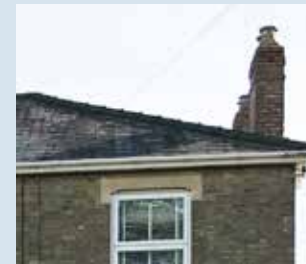
Hipped roof with chimney stacks
