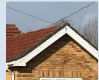
Pitched roof with pantile
