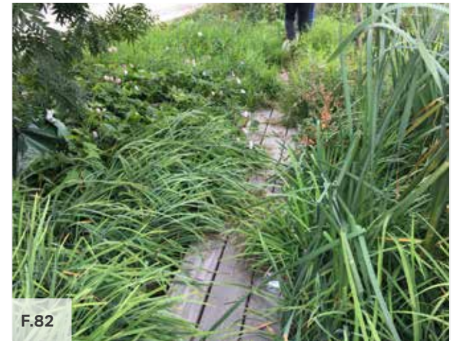
Figure 82: Examples of SuDS designed as a public amenity and fully integrated into the design of the public realm, Sweden
