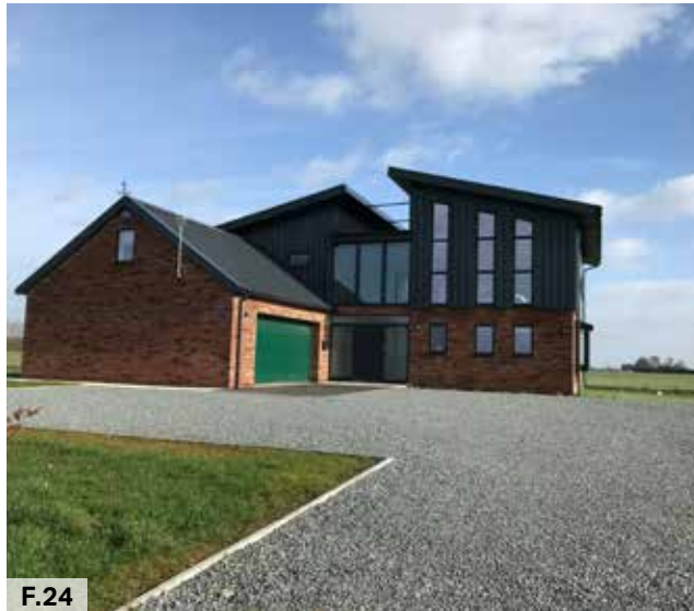
Figure 24: Modern two-storey building on Moyses's Bank with shed roof style and mix of red brick and weatherboarding
