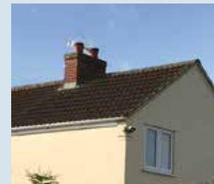
Chimney stack with glazed pantile
