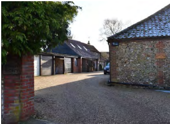
Figure 6- Converted historic agricultural buildings set behind the building line along The Street
