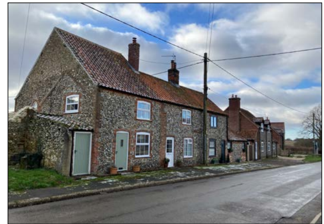
Figure 04: Flint terraces on Docking Road.
