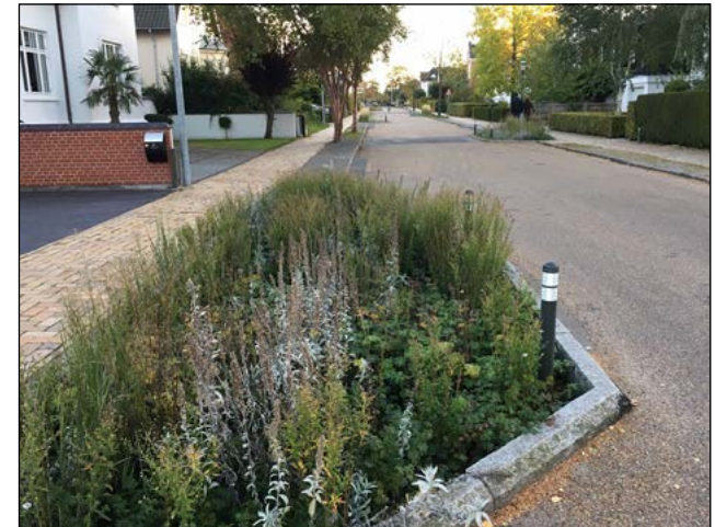
Figure 30: Kerb build-outs that incorporate landscaping and signs could form gateway treatments (source: Cycling Embassy of Denmark).
