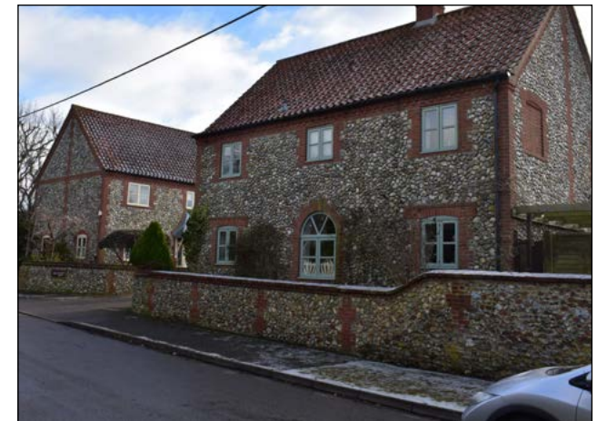
Figure 50: Example of an attractive boundary wall making use of vernacular red brick and flint.
