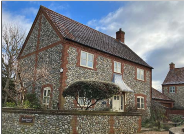
Figure 22: Local example of a contemporary two-storey detached dwelling with a cobblestone exterior finish and red brick detailing.
