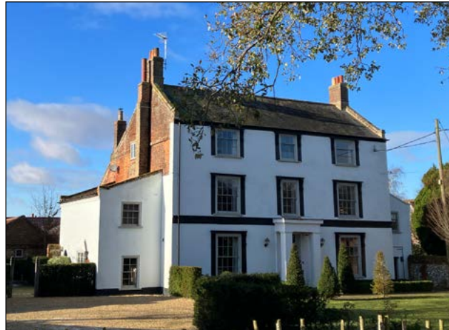
Figure 23: The Manor Farmhouse, featuring a white render exterior finish, with red brick dressing. Large sash windows with glazing bars are also a dominant feature with black decorative lintels.
