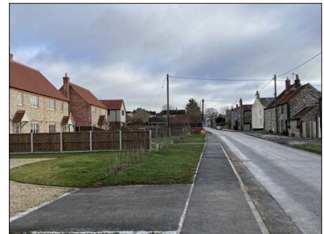
Figure 29: Paths along Docking Road introduced to service new housing development. Pavement a more substantial width of at least 1.8m also featuring grass verges.
