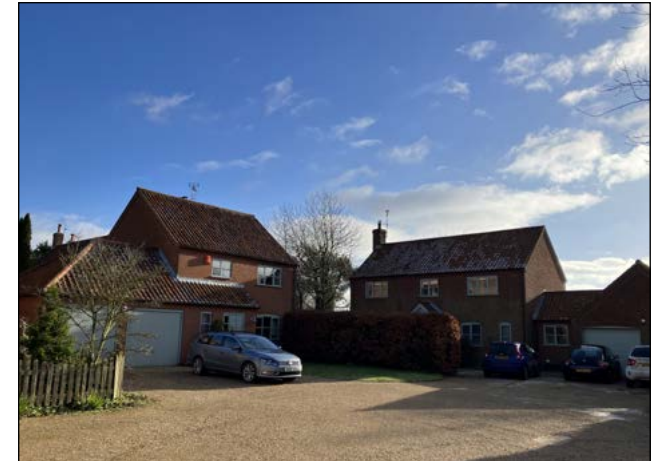
Figure 17: Building set within a small cluster of back-land development set behind The Street.
