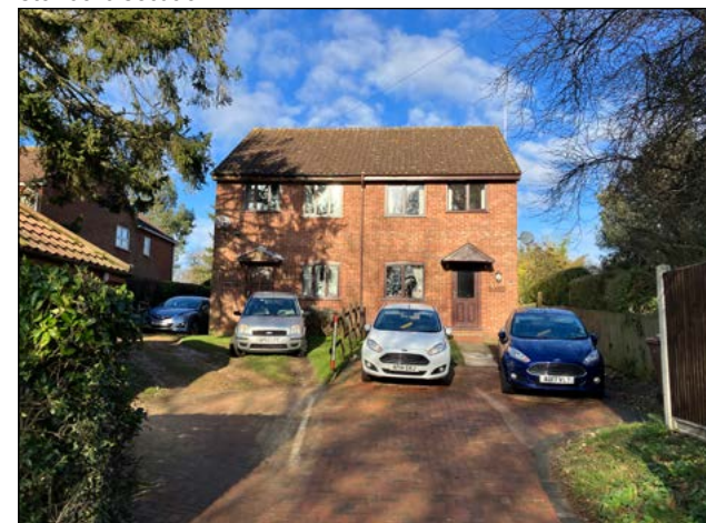
Figure 64: Example of on-plot parking to the front of the dwelling.
