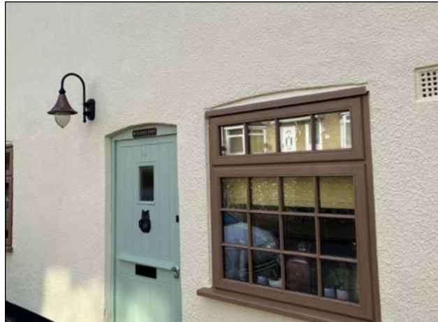
Figure 42: Modern uPVC fenestration applied to older buildings with colour palettes sensitively contributing to the historic vernacular.
