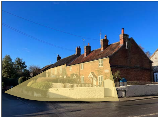
Figure 33: Positive relationship between building fronts and the street enabling views of the pavements and natural surveillance.
