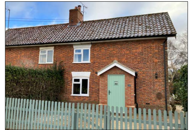
Figure 02: Redbrick semi-detached property on Rudham Road.
