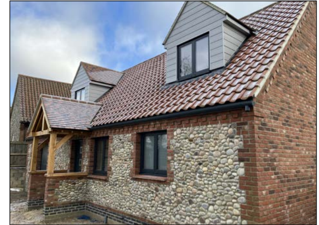
Figure 40: Chalet style dwelling with cobblestone and red brick facade, exposed timber framed porch and pitched dormers
