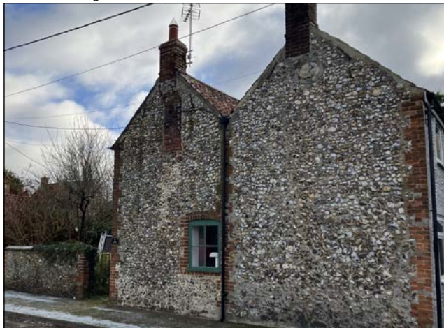
Figure 24: Historic building along The Street with a flint exterior finish with teal casement windows with glazing bars. A typical example of the vernacular within Syderstone's village core.
