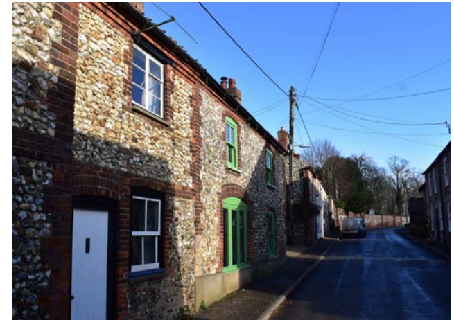
Figure 60: Two storey 19th century terraces on The Street with red brick detailing and flint facades.
