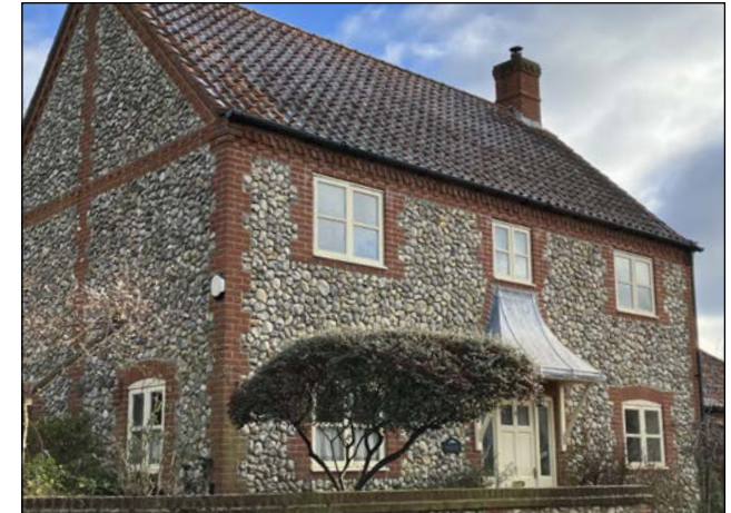
Figure 44: Cobblestones and red brick detailing is a common facade treatment on recently constructed dwellings and contribute positively to Syderstone's prevailing vernacular.
