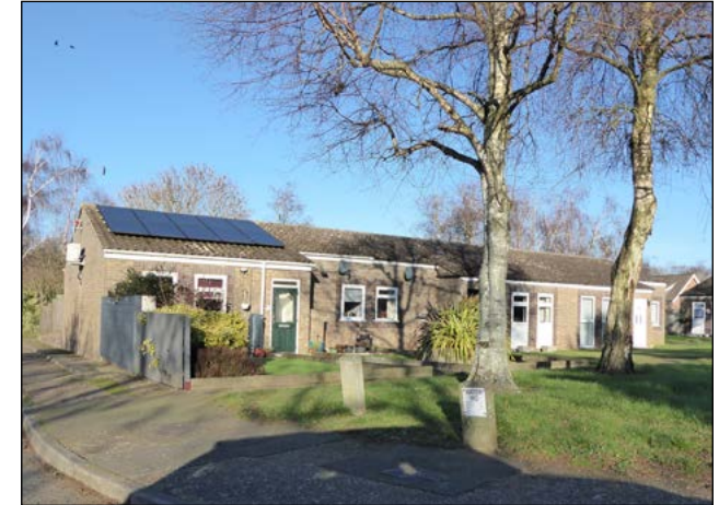
Figure 69: Single storey dwellings at Norman Road.
