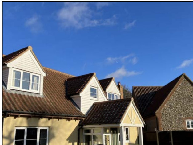
Figure 43: Example of how a mix of contrasting materials between dwellings can positively enhance the overall vernacular.
