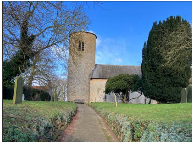
Figure 13: Church of St Mary with round steeple tower.
