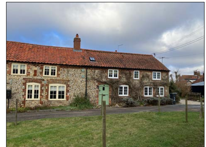
Figure 51: Example of green space on Rudham Road which is framed by a row of 19th century cottages.
