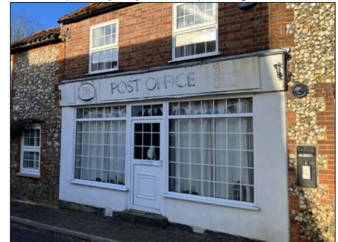
Figure 45: Opportunity to preserve now defunct features such as shop fascias to retain Syderstone's vibrant character.
