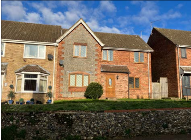
Figure 65: Semi detached house with cobblestone tile facade treatment along the northern edge of The Street.
