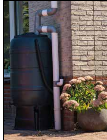
Figure 70: Rain water harvesting with overflow prevention system. (Photo © Milos-Shutterstock 2022)
