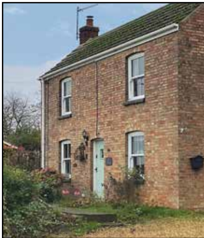
F.26: Traditional sash window and timber door. (Photo © AECOM 2022)
