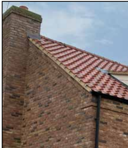
F.33: Red clay tiles and mixed brick. (Photo © AECOM 2022)
