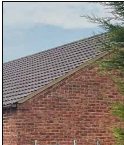
F.34: Clay tiles. (Photo © AECOM 2022)
