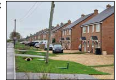
Figure 61: New builds with open swales marking the boundary. (Photo © AECOM 2022)
