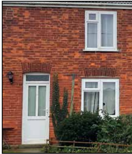
F.30: Red brick. (Photo © AECOM 2022)
