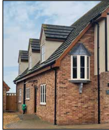
F.25: Dormer and feature window. (Photo © AECOM 2022)
