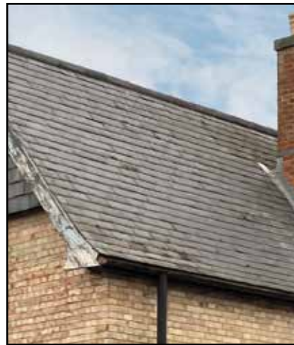
F.35: Slate roof. (Photo © AECOM 2022)
