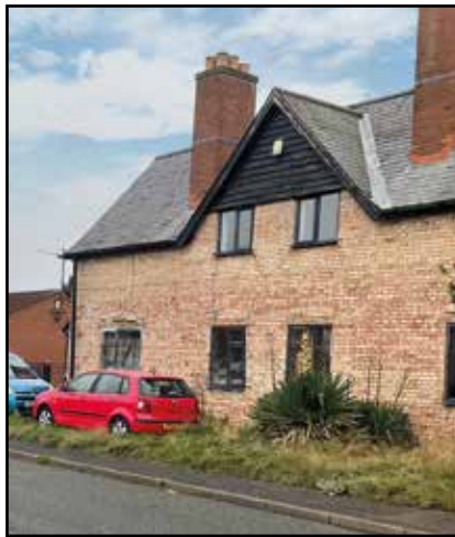
F.28: Over sized chimney stacks. (Photo © AECOM 2022)
