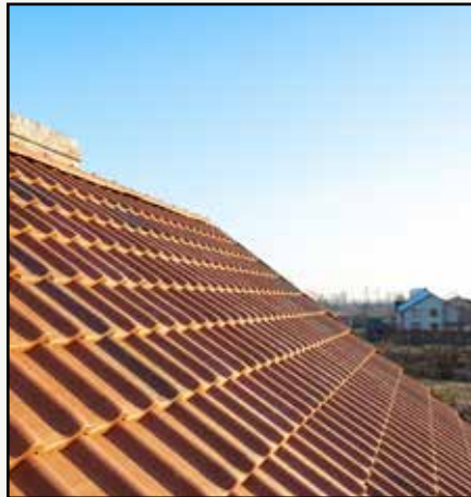
F.56: Quality, red clay tile roof (Photo © Adobe Stock 2022)
