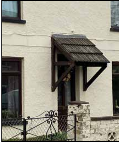
F.24: Covered porch older style. (Photo © AECOM 2022)
