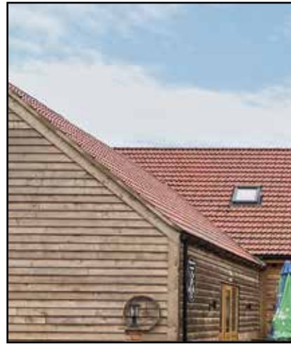
F.32: Wood cladding. (Photo © AECOM 2022)
