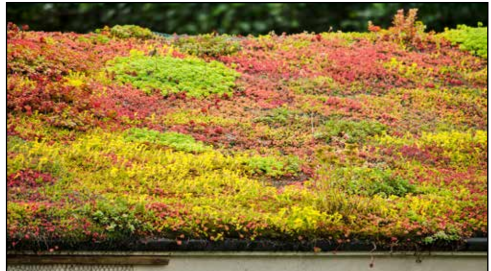
Figure 94: Natural flood prevention, green roof as part of a SuDS management system.
