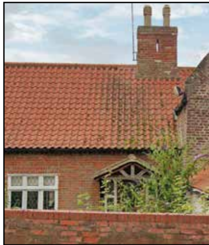
F.41: Covered porch on period property. (Photo © Google Earth 2022)
