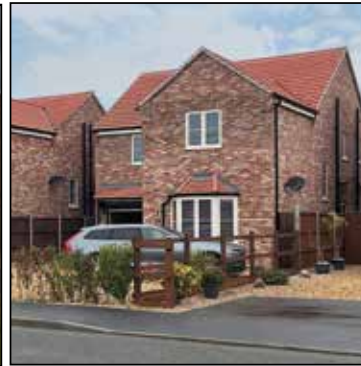
Figure 82: Example of front parking with screening. (Photo © AECOM 2022)
