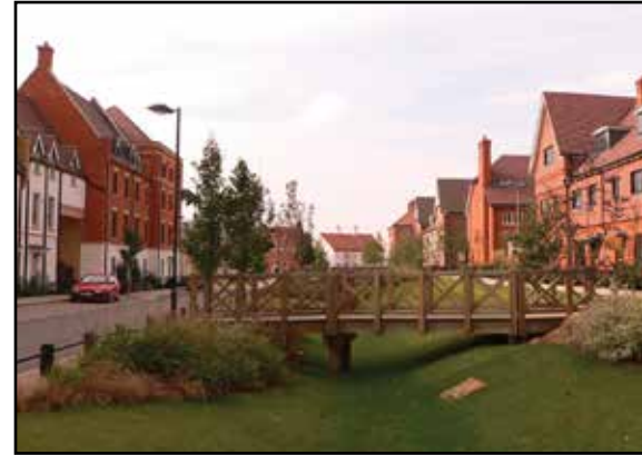
Figure 88: Example of open drainage channels. (Photo © AECOM 2022)
