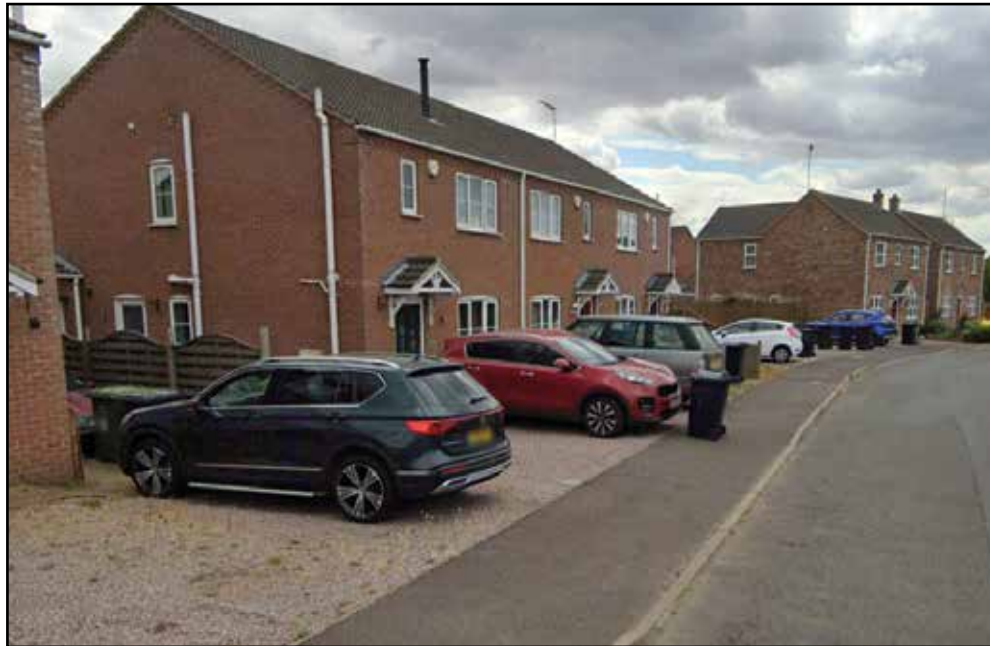
F.58: Example of cramped on plot parking with no screening. (Photo © Google Earth 2022)
