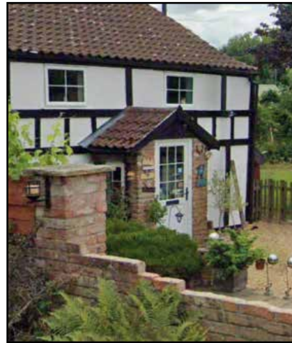
F.42: Render and half-timbered styling on cottage. (Photo © Google Earth 2022)
