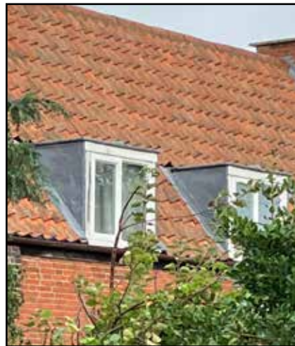
F.44: Dormer windows. (Photo © AECOM 2022)
