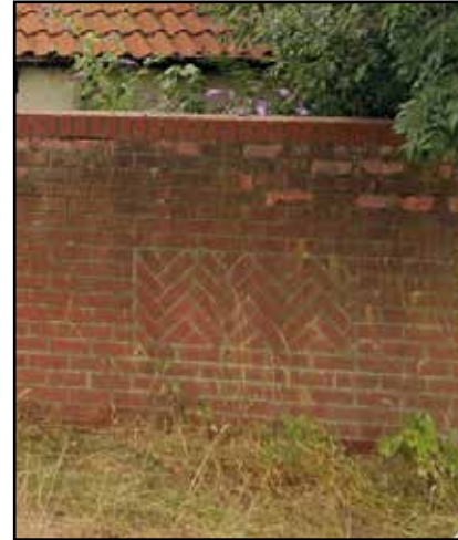
F.48: Red brick detailing on wall. (Photo © AECOM 2022)
