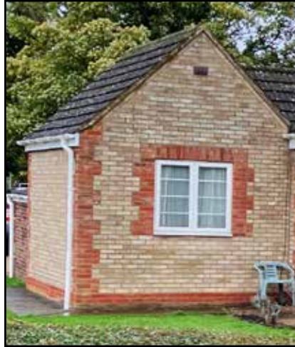
F.47: Mix of Red brick and white brick on the Alms Houses adjacent to St. Andrew's Church. (Photo © AECOM 2022)
